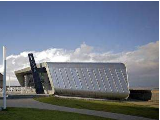
New Café and Toilets at West End Gardens
